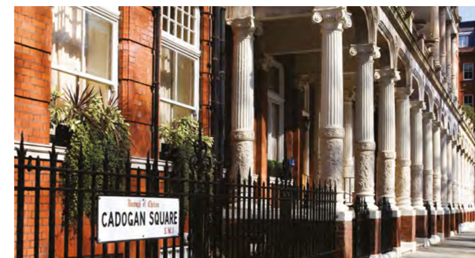
← The Places Management team ensures properties are well maintained. ↓ Cadogan Square, Chelsea.
